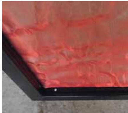
Frame cladding with h-Profile. Prefabricated with PVC flat keder
